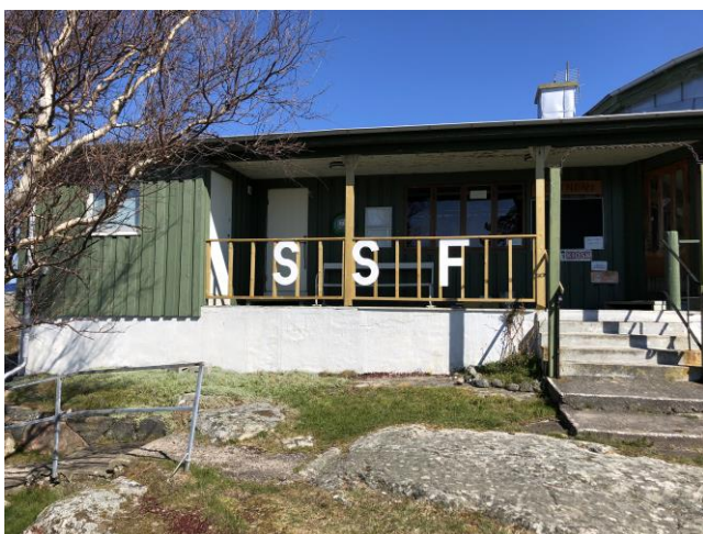
Entrén under reovering
